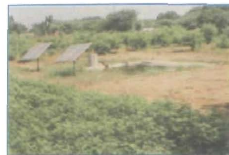
Solar PV panel
