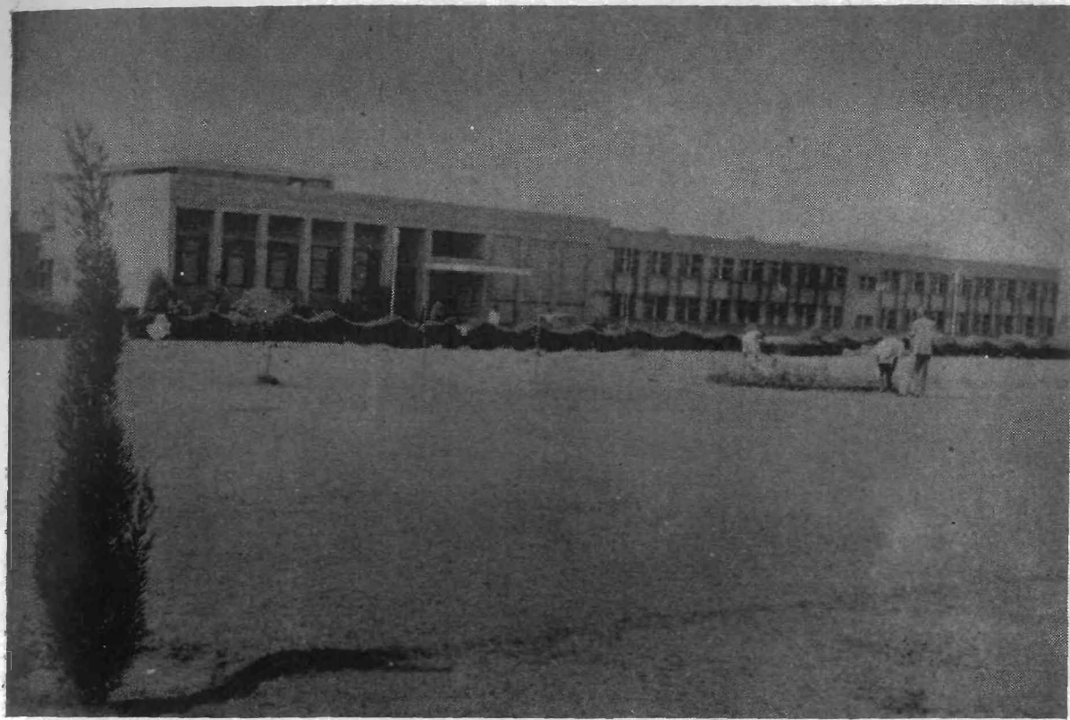
Main Laboratory building, CAZRI
