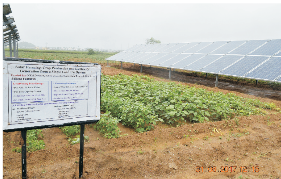
Fig. 25. A view of solar photo-voltaic system of 25 KW capacity along with crops between and beneath panels
