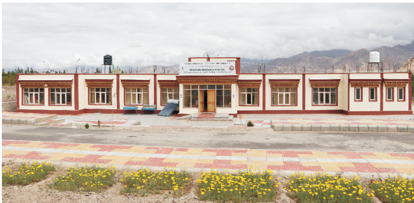
ICAR-CAZRI-RRS-Leh office building
