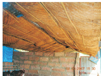
Thick thatched panel under the asbestos roof reduces thermal stress
