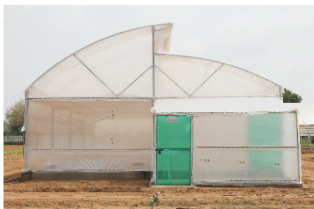
Naturally ventilated polyhouse
