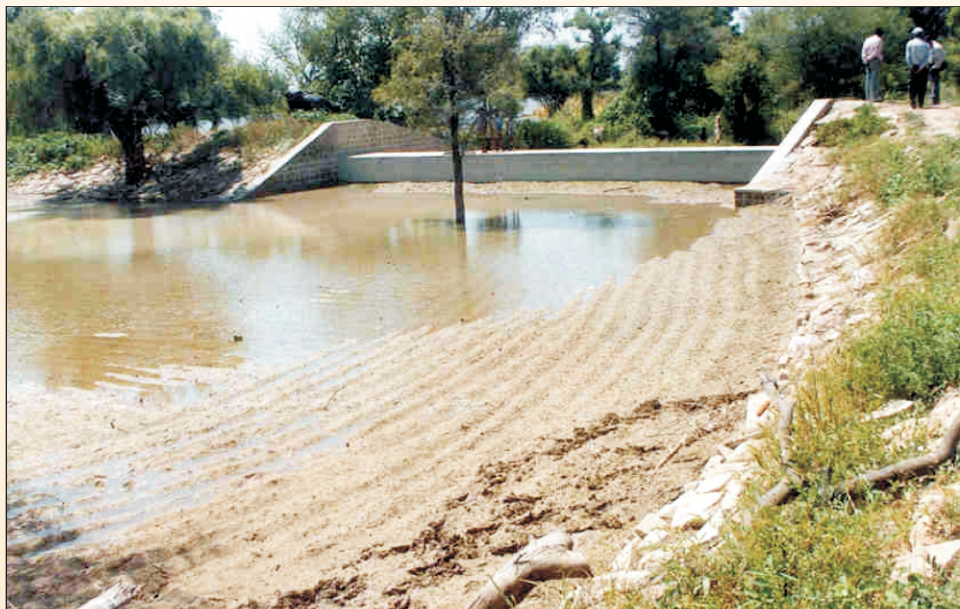
Fig-11. Khadin with wastewier at Baorali-Bambore watershed (Jodhpur)
