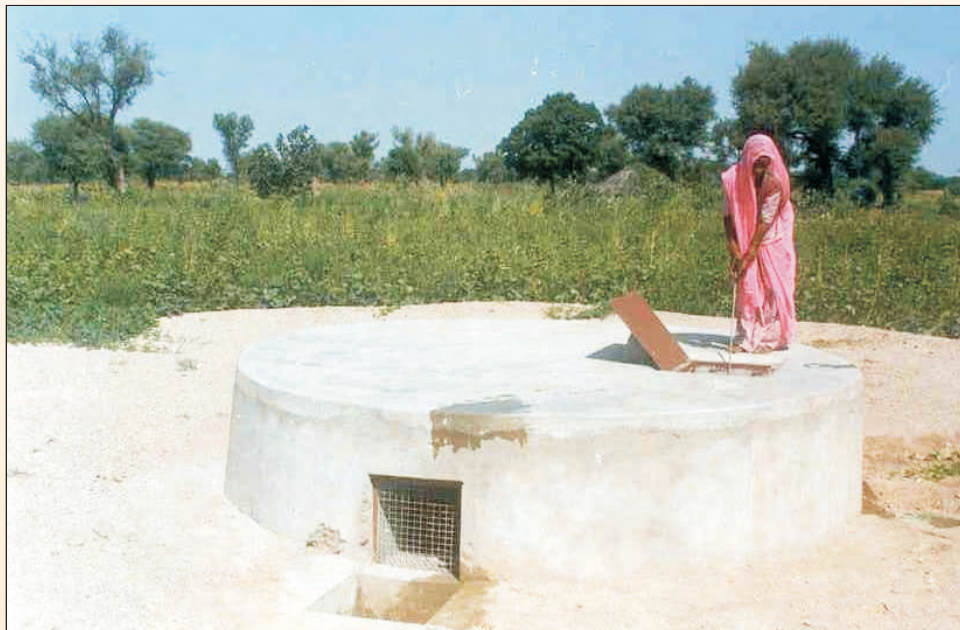
Fig-9. Improved tanka of 21 m 3 capacity at Baorali village (Jodhpur district)
