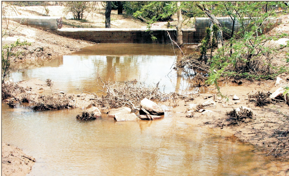
Fig-7. Check-dam at Beriganga research farm of CAZRI, Jodhpur
