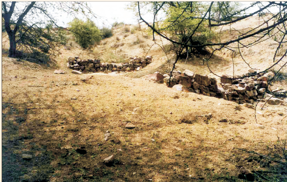
Fig-8. A series of Loose stone check-dams (LSCD) at gully in Jhanwar Watershed (Jodhpur)
