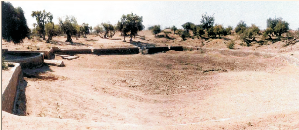
Fig-10. Improved nadi with inlet and outlet
