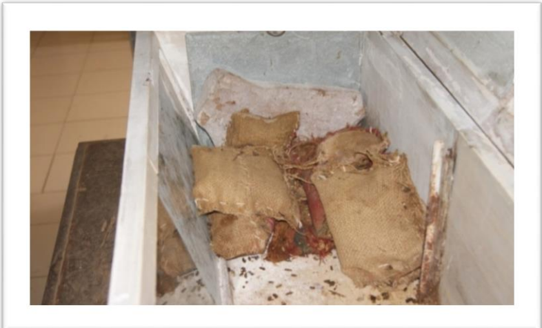
Gunny bags stacked in the area with walls and floor applied with 3% Ziram Solution
