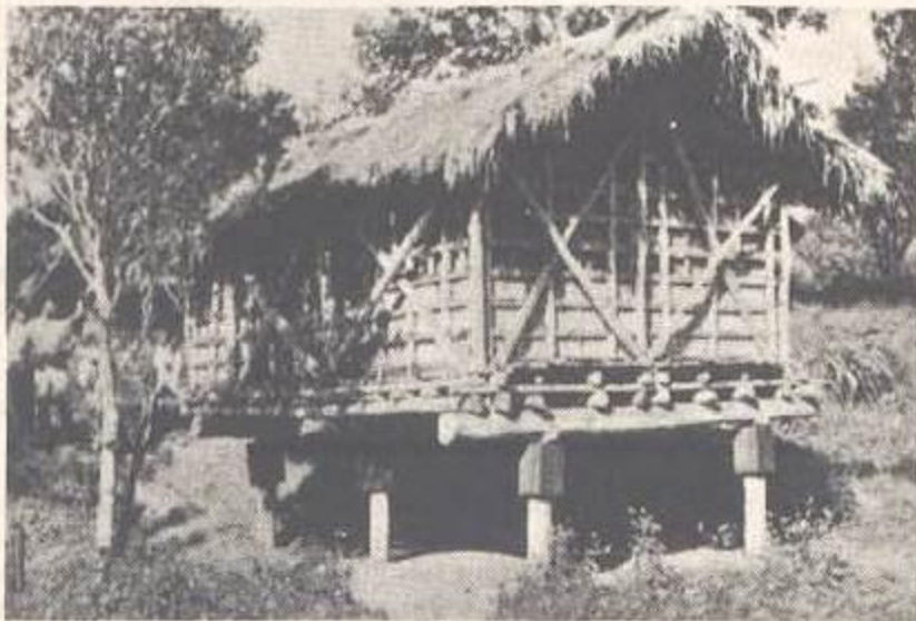
Fig 1 Rodent proof storage structure in rural areas of Arunachal Pradesh
